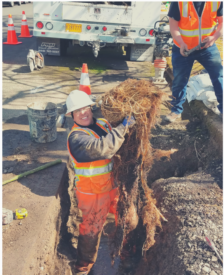
Arturo Madrid poses with his prize - a massive root mass he and his team removed from a storm line on Latona Drive NE this spring.
